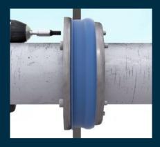
Fit the seal against the inside of the opening and tighten the bolts. It maintains a tight seal around the pipe and inside the opening.
