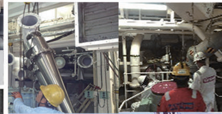
Ship Owner □ Germany (CP Offen) | Ship Type □ 4100TEU Container Pump Capacity □ 500m 3 / h x 2 | Model □ BSKY500 x 1 set Skid Type Class □ GL
