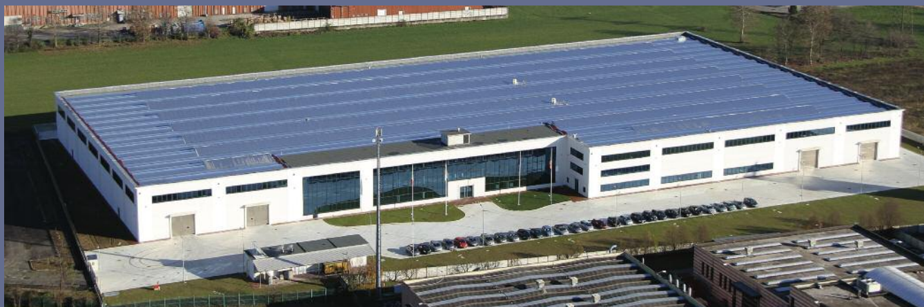
Filtrex Manufacturing Unit #4 - 22,000 covered sqmt - Vignate (Italy)
